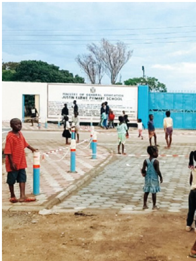
Justin Kabwe Primary School Lusaka, Zambia, 2017
